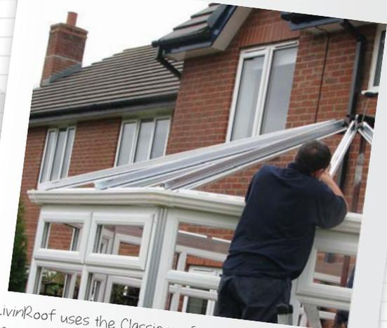
LivinRoof uses the Classic roof system so fitters can swap an old for a new one very quickly
